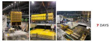
Completion of formworks, reinforcement and connection between blocks and final casting:
